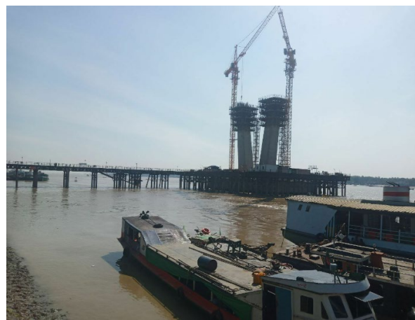
Yangon-Dala River Bridge under construction.
