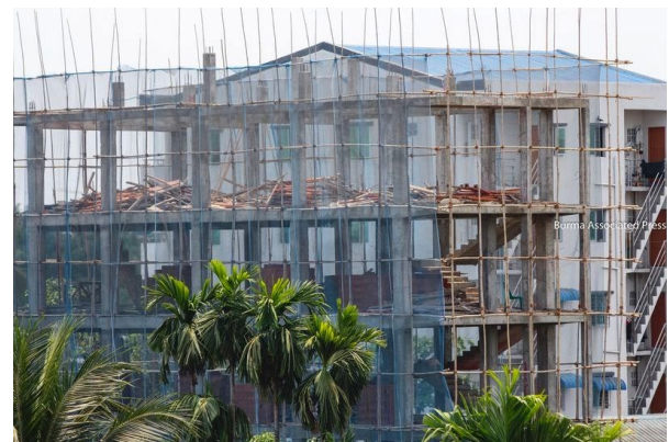
A building under construction stage.
